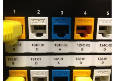
and termination. Patch panel labeling will be done mechanically and the labeling font size will be 18 point, (3/16"). Patch panel ports 1-12 & 25-36 will terminate on switch ports 1-24 and patch panel ports 13-24 & 37-48 will terminate on switch ports 25-48.
